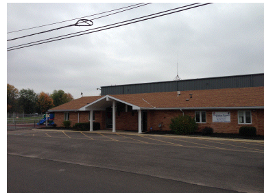
Dawsett Center – Crawford County Head Start Center 525 Dawsett St. Gallion, OH 44833
