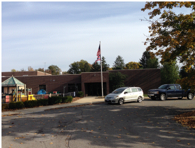
Mt. Gilead Head Start Center (Whetstone Building) 406 Banks St. Mt. Gilead, OH 43338
