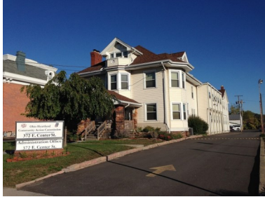
Administrative Office 372 E. Center St. Marion, OH 43302
